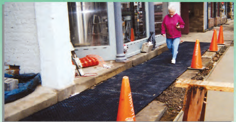
VersaMATS lock together to form continuous walkway
